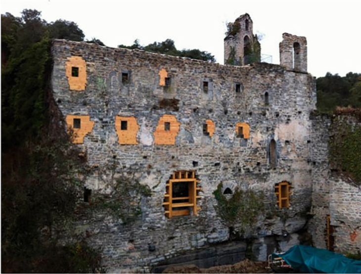
Fig. 2 Santa Catalina de Badaya (SP) restored by isuuru architects (Source: http://isuuru.com/pat_consolidacion.html . Accessed 29 Jan 2022): Restored ruin with clearly contrasted wooden additions and less visible consolidations (Photo: © isuuruarquitectos)
